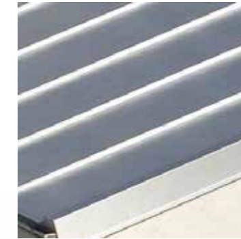
Aluminium standing seam roof in anthracite grey
