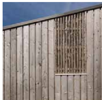
Larch timber cladding
